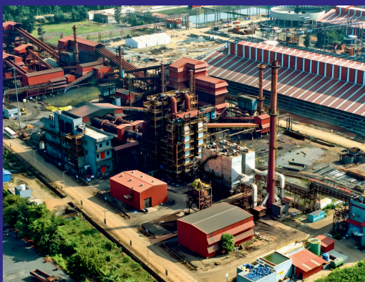
Waste Heat Recovery Boiler based 5 MW Power Plant for Lloyds Metal And Energy Limited, Konsari
